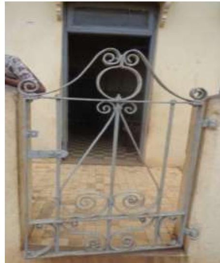
Plate 2. Aganrandi , (metal fabrication and coupled with bolts and nuts), at the open entrance of old Ota palace. (Photograph by Sobowale T.O., 2014
